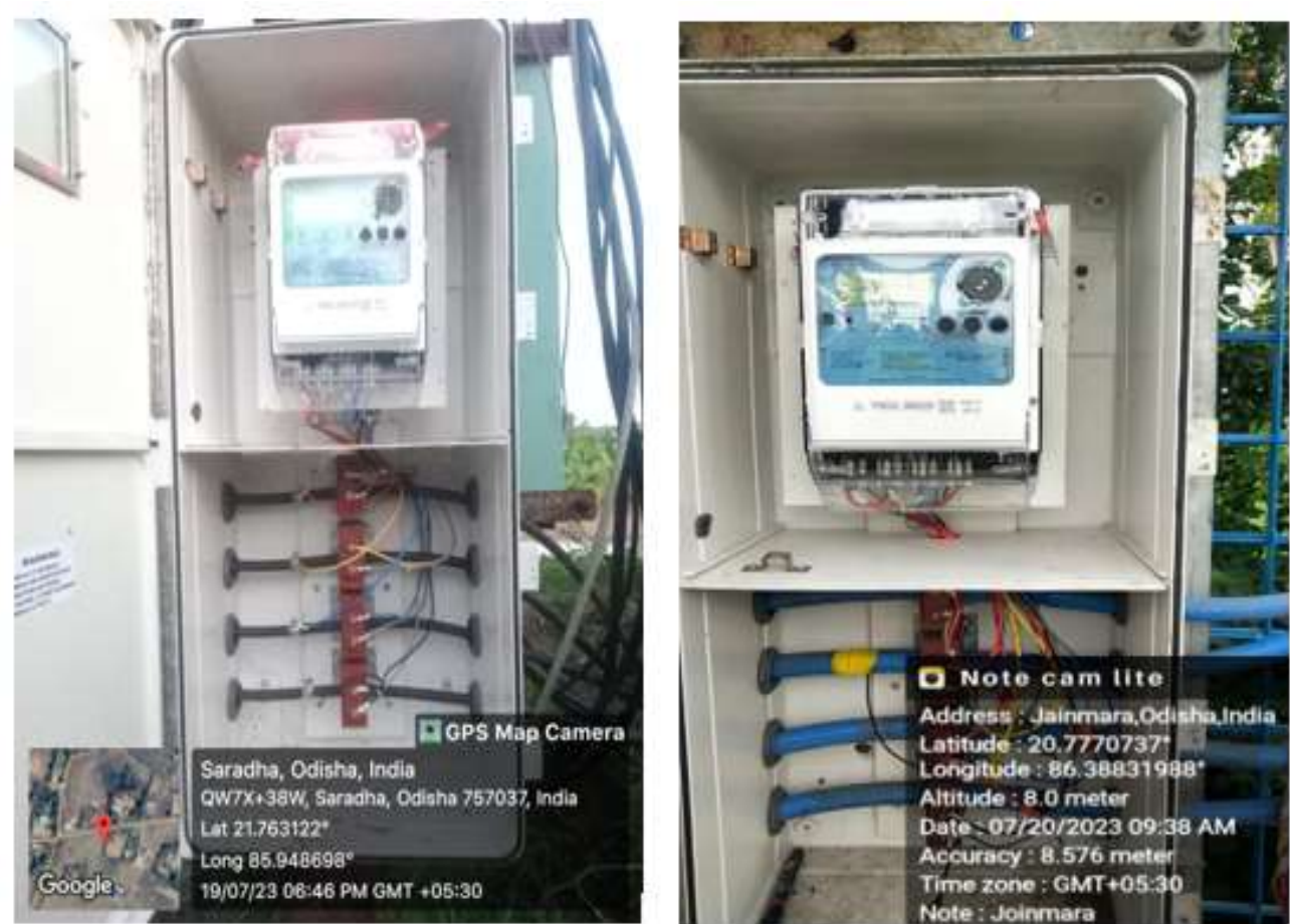
SAMPLE PHOTOGRAPHS OF DT SMART METER INSTALLATION
