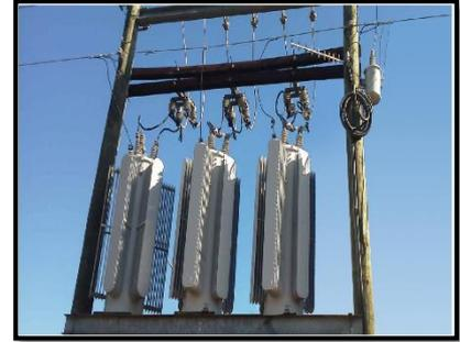
Figure 1: Pole mounted voltage regulator installed in a distribution network
